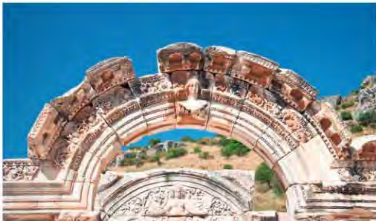
■ Figure D4.2.7 An arch from the Temple of Hadrian, Ephesus, Turkey. The keystone (the central stone) supports the arch – without it the arch would collapse
